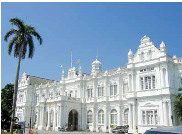
The Penang City Hall building will undergo refurbishment works.
